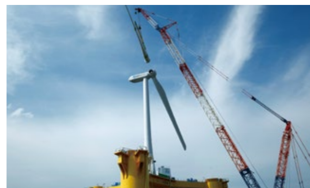
The wind turbine was mounted at the MES Chiba Works and towed to the Onahama Bay in Fukushima Prefecture.
