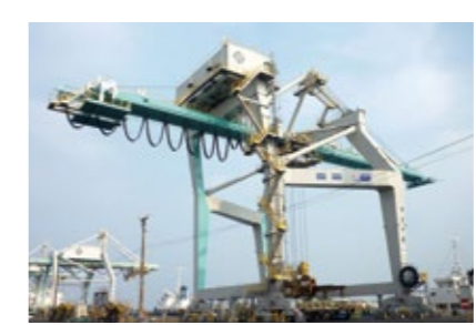
Bridge Type Crane for Shipment of Products
