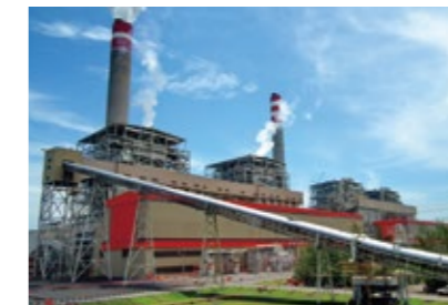
Marine and Land Public Work for Coal Fired Power Station "TANJUNG JATI"
